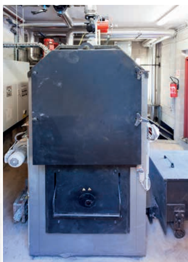
Chaudière C.E.L., 220 kW
